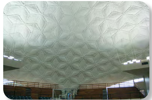
Acoustic ceiling application, A.E. Wood Coliseum, Clinton, MS
