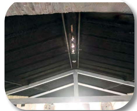
Charcoal tinted Sonoglass Acoustic Insulation, applied to restaurant ceiling, NY.
