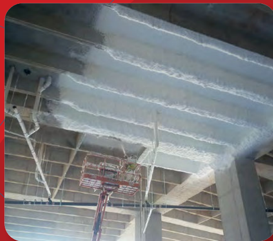
U.S. Bank Stadium, Minneapolis. Irregular surfaces easily insulated with Monoglass Spray-On.
